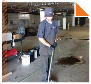
**Problem:** An old apartment building in Valencia, California, needed to be gutted and redone. The inspection of the plumbing system determined that the main drainpipe leading to the city sewer system out of the building was buried 5 feet below the concrete floor of the parking garage. While breaking the floor was an option, the cost of doing so was out of the budget. The 8-inch line ran the entire 110 feet of the structure.
